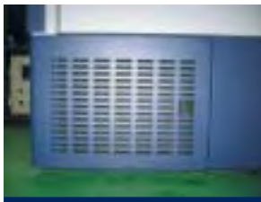
Filters are detachable and easily accessible through a condenser door. This makes cleaning the air filter a quick and easy job.
